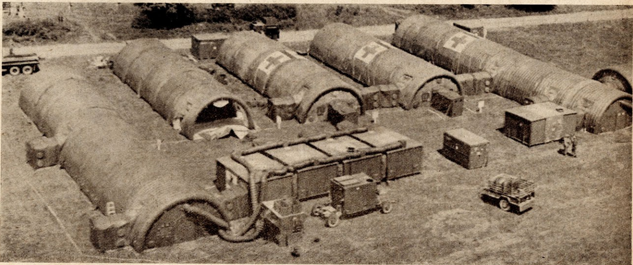
This aerial view shows the final stages of inflating the 32nd Surgical Field Hospital at the training site. This hospital is composed of inflatable units designed to be set up in a few hours to provide medical treatment.
